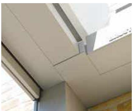
Water drainage through the gutters directly into the supporting posts
